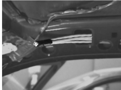
Cable bundle exiting passenger-side cable exit opening
