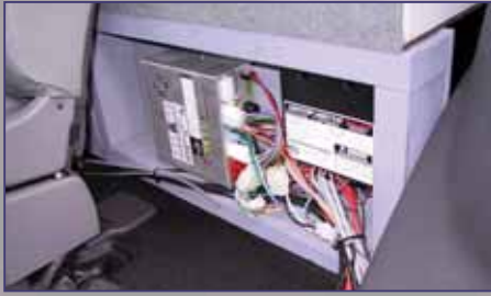
CSP660 installation with CenCom™ amplifier.
