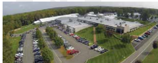
Chester, Connecticut facility
